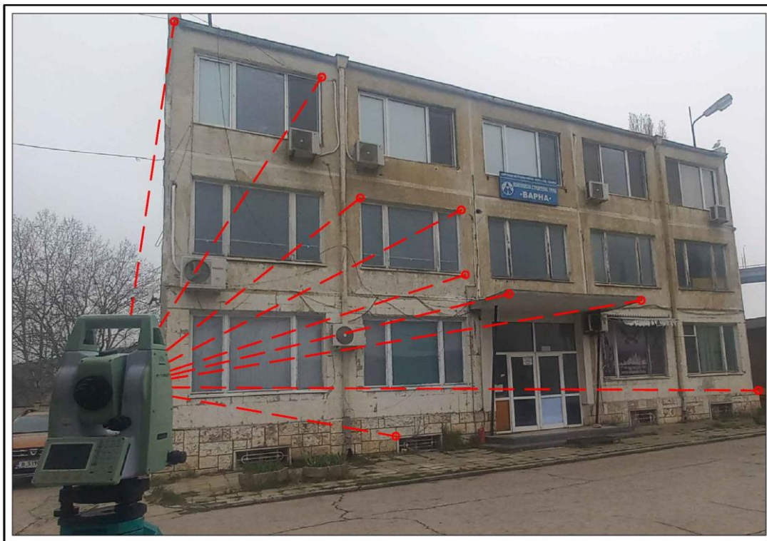
Fig. 1. Geodetic survey of a facade
