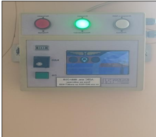
Fig. 5. Automatic Crossing Device (APU) Panel
